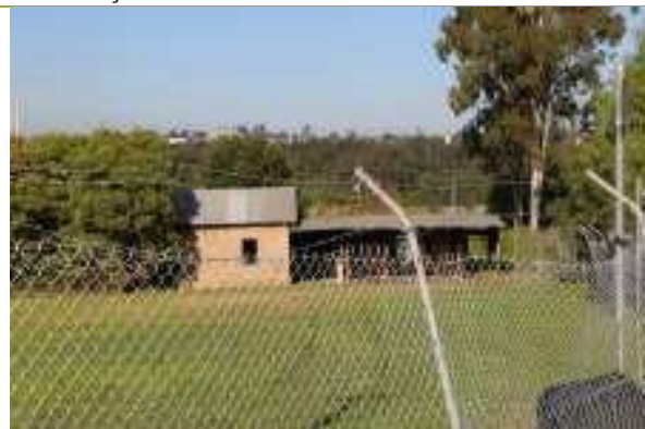
Fence and ancillary structures.
