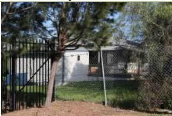
Fence and ancillary structures.
