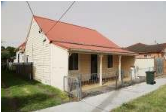
22 New York Street, front façade.
