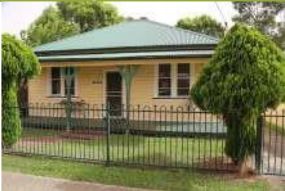
13 New York Street, front façade.
