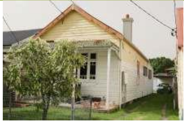
20 New York Street, front façade.
