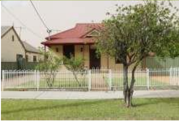
14 New York Street, front façade.
