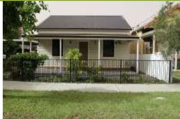
18 New York Street, front façade.
