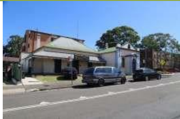
View from Mary Street to front façade of the Former Bank and Residence.
