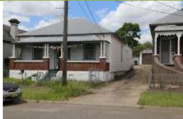
View from Hewlett Street to the west elevation and driveway between 8 Hewlett Street.
