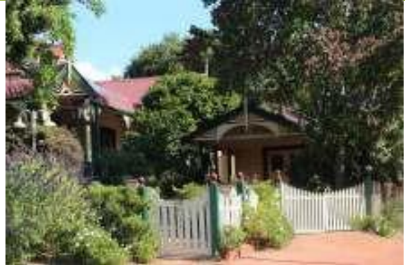
Detail of front façade, carport, fence and landscaping.
