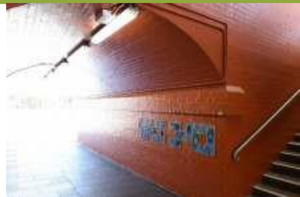
Tunnel under Berala Railway Station.
