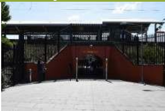
Entrance tunnel to Berala Railway Station.
