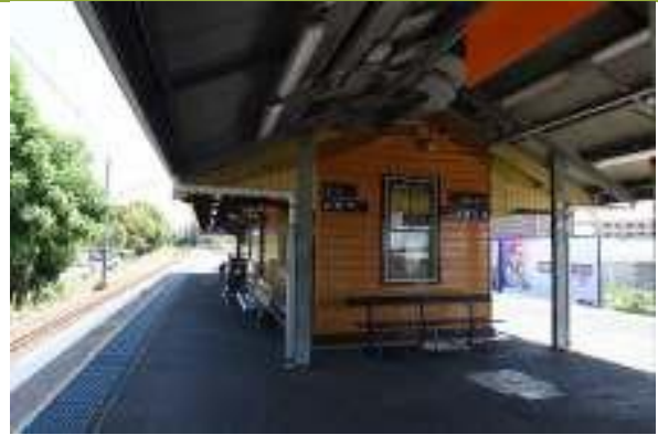
View to Platform 1 and 2.
