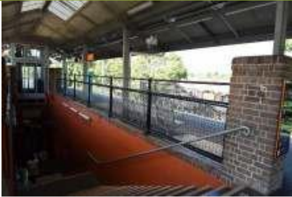
View to Platform.
