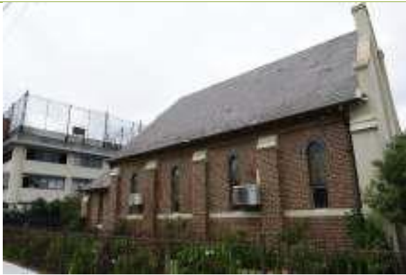
Side elevation of Uniting Church.
