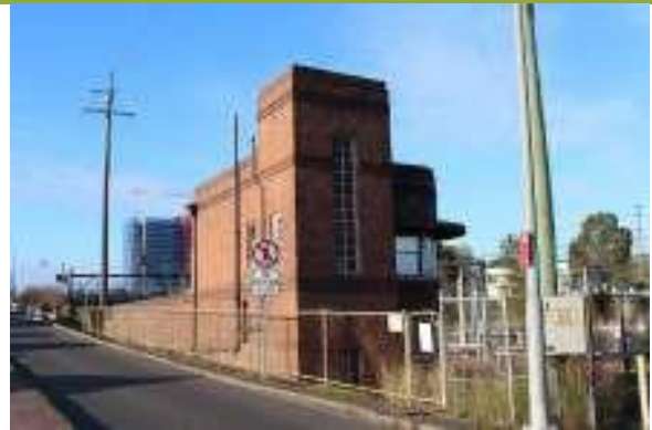
View to north-western and north-eastern elevations of Signal Box
