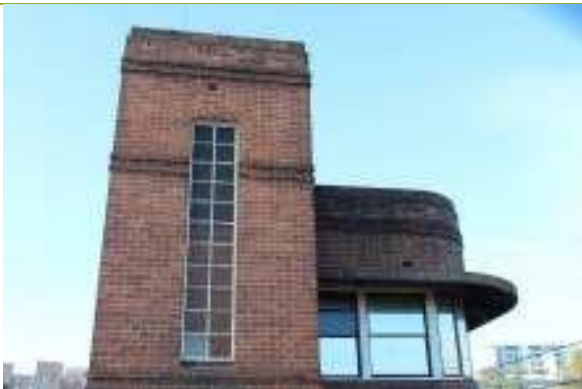
Detail of north-western elevation of Signal Box.
