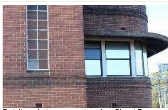
Detail to windows as replaced on Signal Box.
