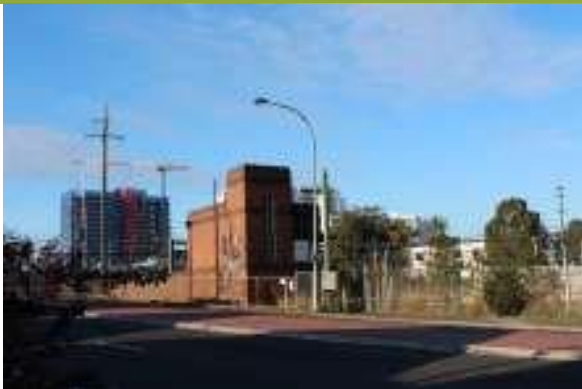
View to Signal Box from Rawson Street.
