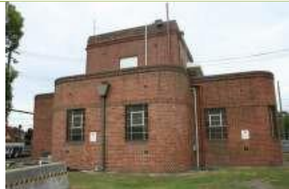
View to Clyde Signal Box.
