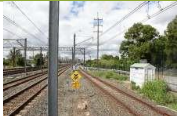
Overview of Clyde Marshalling Yards.
