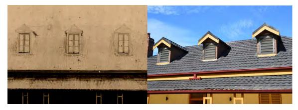
Figure 2.7 I Window sashes in the dormers, circa 1905, which were probably casement sashes. (left); louvres in dormers, 2021 (right).
