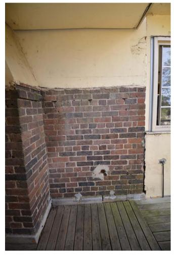
Figure 2.12 | Brickwork on the southern side of the southern wings (Rooms 6 and 7) requires repairs to mortar, replacement of new bricks where holes have been formed and careful removal of cement patching.
