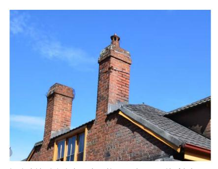
Figure 2.10 I Deteriorating brick pointing in the northern chimney on the eastern side of the house.
