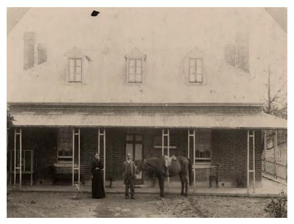
Figure 2.21 Photograph of "The Wattles", circa 1905, showing corrugated iron on the main roof and the configuration of the front door and windows. [Reproduced in Rosemary Broomham, *The Wattles: A History*]
