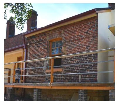
Figure 2.11 I Cracking in the western wall at the rear of the building has been an ongoing problem. Attempts to repair it in the past has been carried out crudely.
