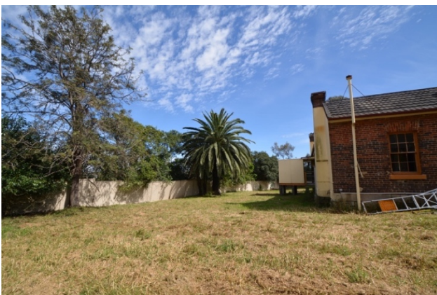
Figure 4.14 | View of rear yard and SE corner of the house.
