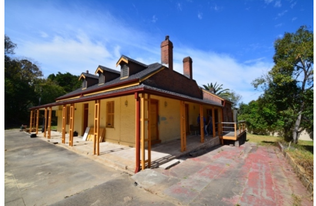
Figure 4.4 | NW corner and western verandah.
