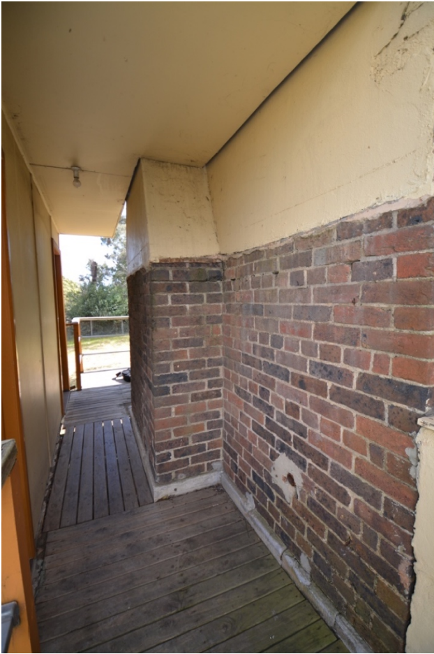
Figure 4.7 | SW side of the rear of The Wattles. Chimney breast and chimney extant.
