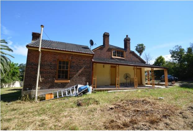
Figure 4.1 | Eastern side of The Wattles .
