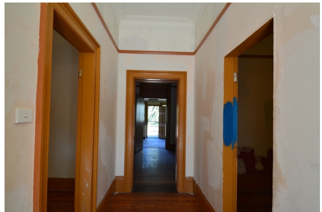
Figure 4.17 | Hallway B with Room A at left and Room C at right.
