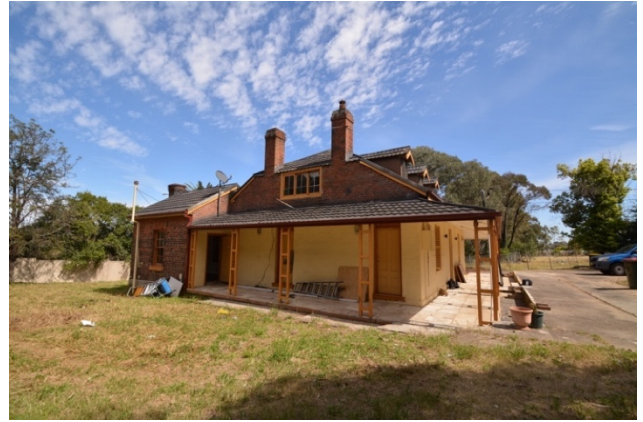
Figure 4.2 | NE corner and side and front verandah.
