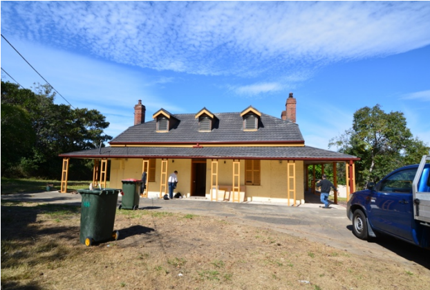
Figure 4.3 | Front (northern elevation) of the study site.
