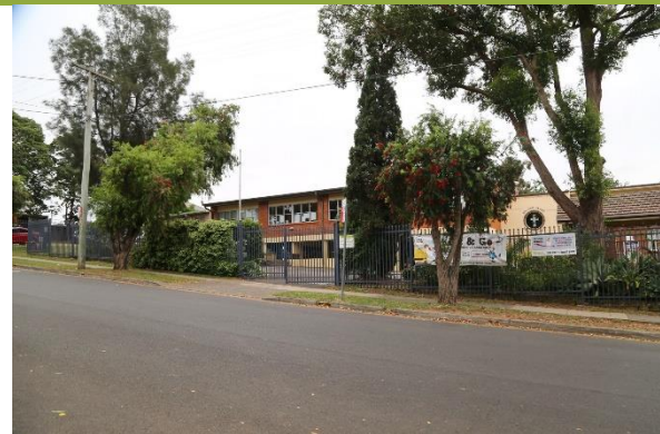
View of School buildings.
