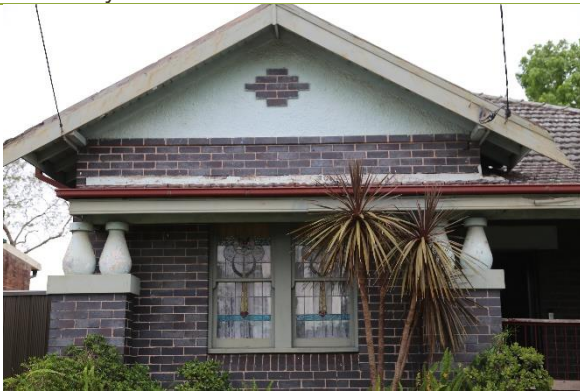
Projecting gable wing.
