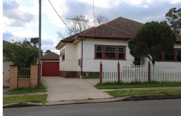
View north from Grand Avenue to garage.
