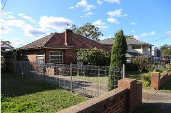
View to 45 Austral Avenue.
