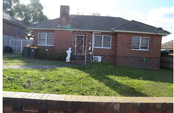
View to 47 Austral Avenue.
