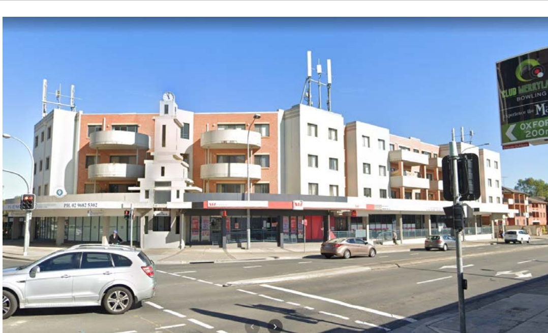
Figure 12 – Shows the 4 storey mixed use buildings to the west of the site, separated by Treves Street
