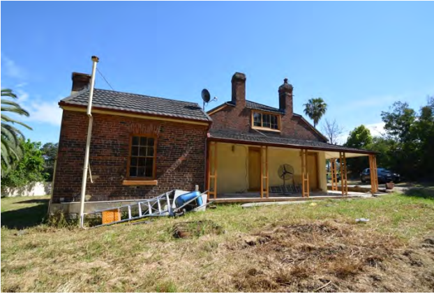
Figure 4.1 | Eastern side of The Wattles .
