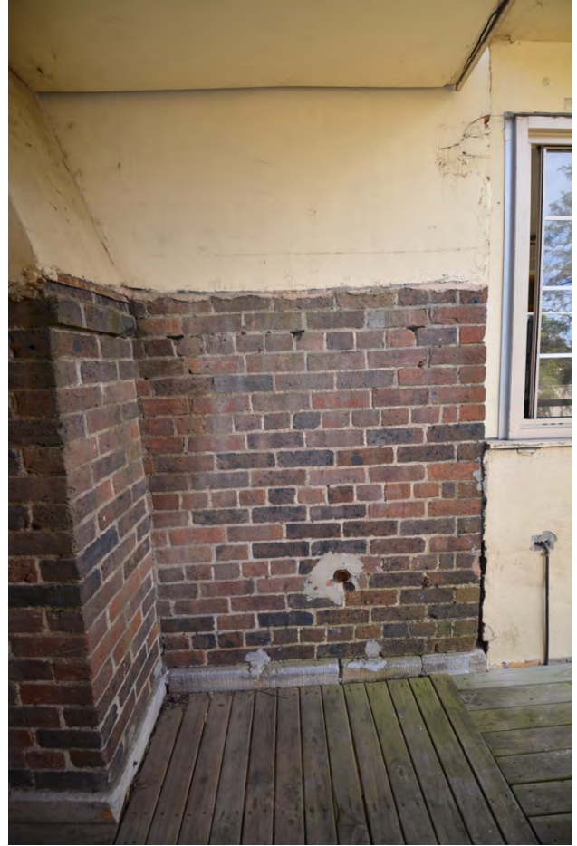
Figure 4.8 | Facebrick on a sandstone base at rear.
