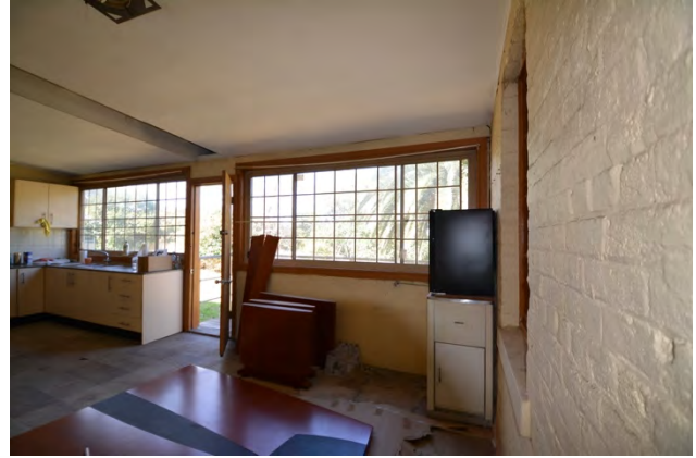
Figure 4.12 | Infilled area at rear (looking SE). Original window extant at right.
