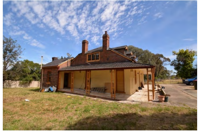
Figure 4.2 | NE corner and side and front verandah.
