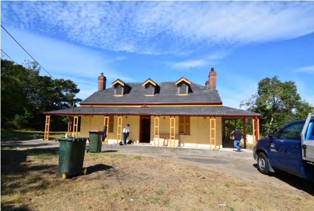
Figure 4.3 | Front (northern elevation) of the study site.
