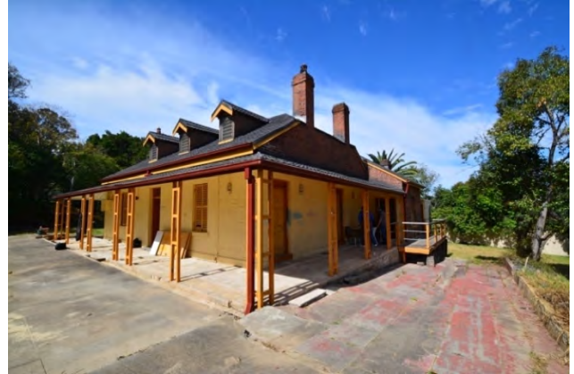
Figure 4.4 | NW corner and western verandah.
