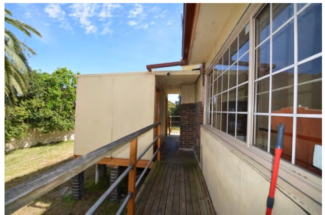
Figure 4.10 | View W along the rear of the residence.
