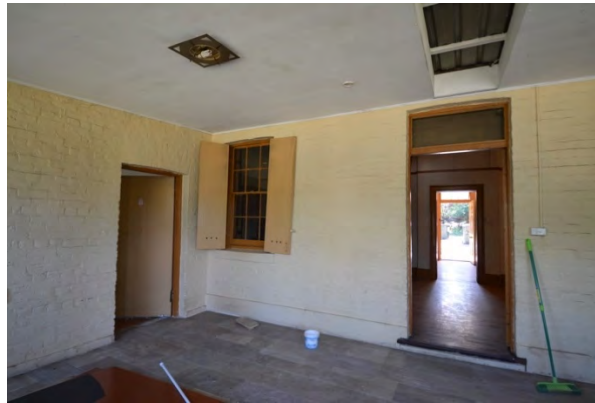
Figure 4.13 | Former exterior rear wall of The Wattles, including rear door. Evident is the central hallway that continues through the house from the front door. This central axis is a significant element of the layout of the house.
