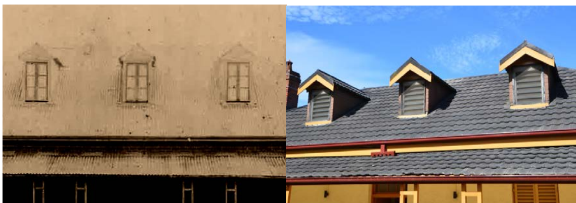
Figure 2.7 | Window sashes in the dormers, circa 1905, which were probably casement sashes. (left); louvres in dormers, 2021 (right).
