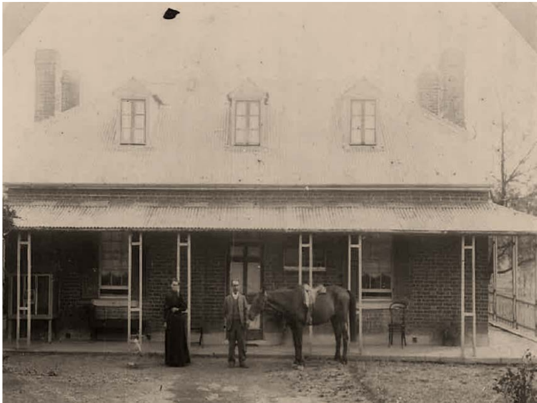
Figure 2.2 | Photograph of "The Wattles", circa 1905, showing corrugated iron on the main roof and the configuration of the front door and windows. [Reproduced in Rosemary Broomham, The Wattles: A History ]
