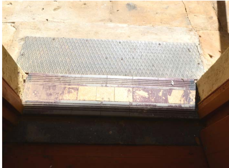
Figure 2.8 | Tiled threshold at the front door.
